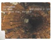
After: the sewer has been fully lined, with any disruption kept to a minimum.
